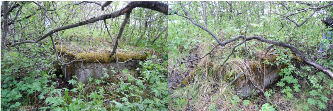
Betongfundament bak brakke 9
